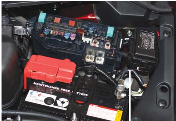
Negative 12-Volt Battery Cable
