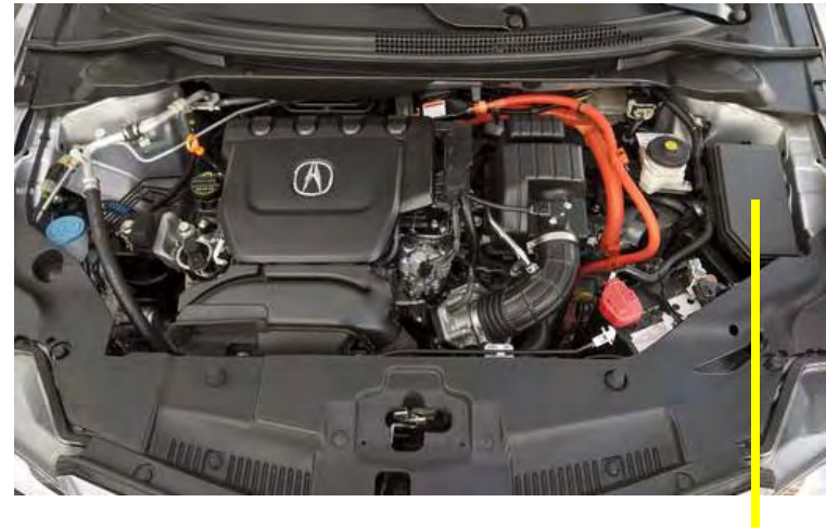
Underhood Fuse Box
